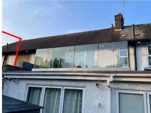
Image 10 Sunlight that will be blocked for more than 3 months of the year (red line location of proposed first floor rear extension).
